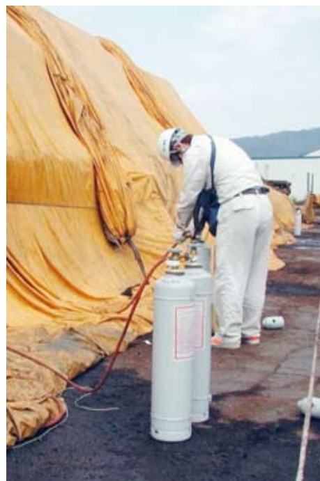
Applying methyl bromide under sheets to imported logs as a quarantine treatment (Ministry of Agriculture, Forestry and Fisheries, Japan)
